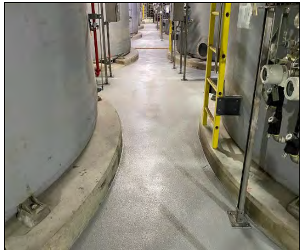
Finished Epoxy Coated Floor
