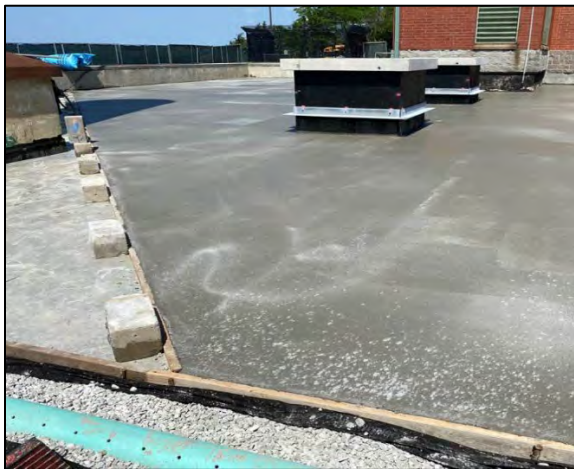
Sloped Concrete Topping Slab
