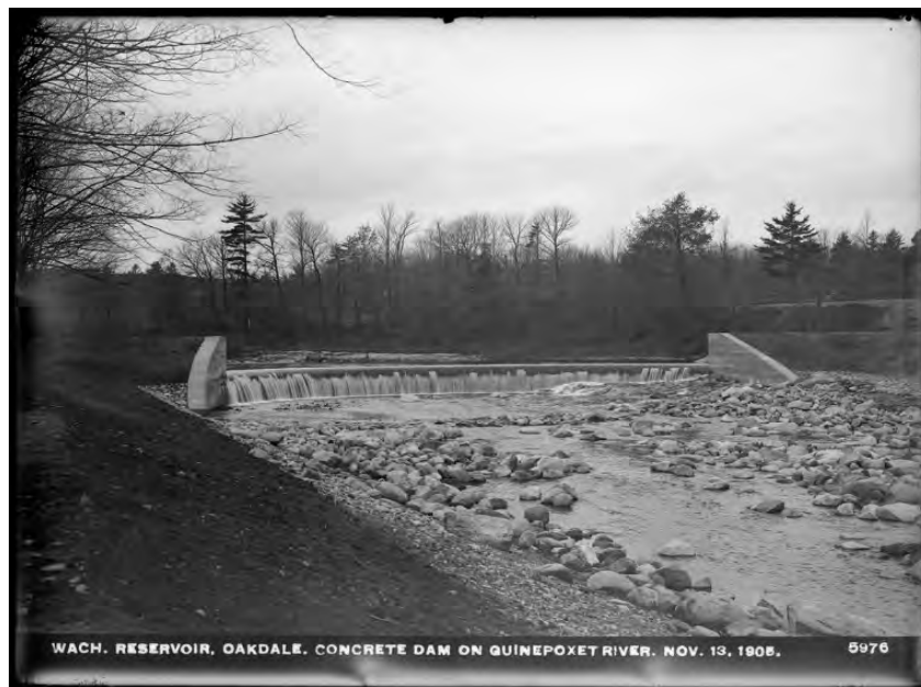
Figure 2. Quinapoxet Dam soon after construction in 1905
