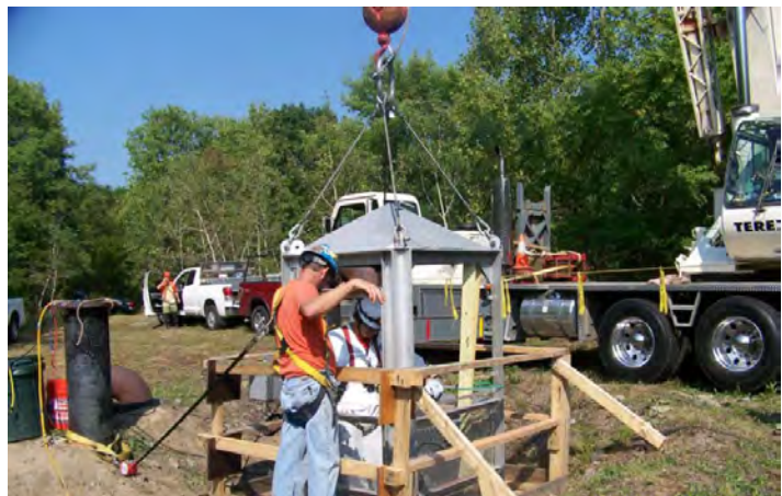
Figure 1: Construction-basket descending at the Construction Shaft
